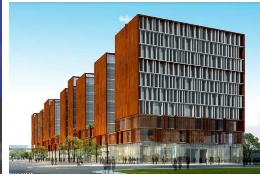
D2, SOHO, Sentul (On-Going)
