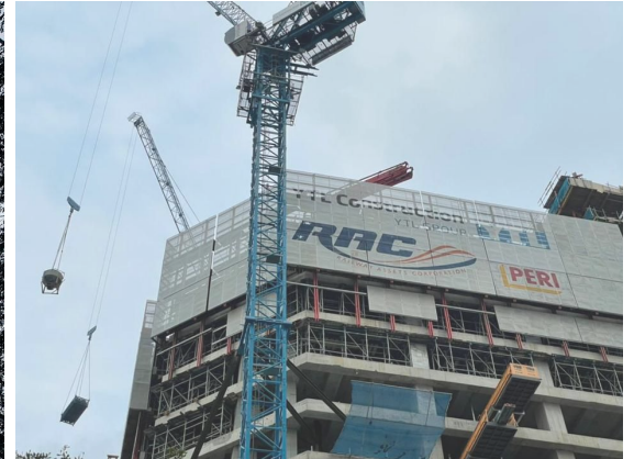
RAC Tower, Brickfields (On-going)
